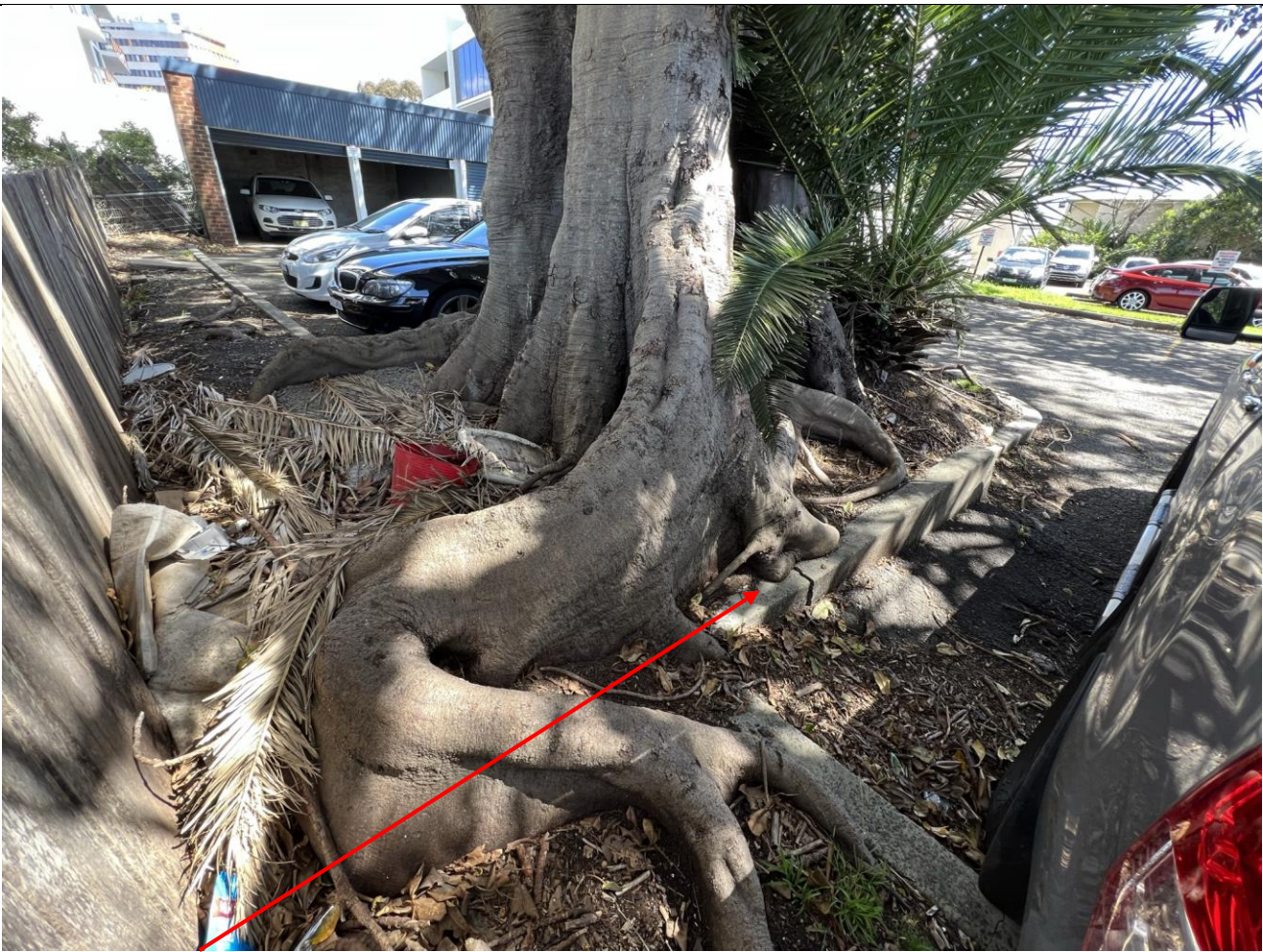
Image f: T6- All this concrete edging must be retained in place or very carefully removed by hand under project arborist supervision
