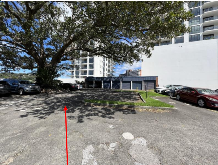
Image g: T6- all this bitumen within a 15m radius of the trunk must be carefully scraped up under project arborist supervision
